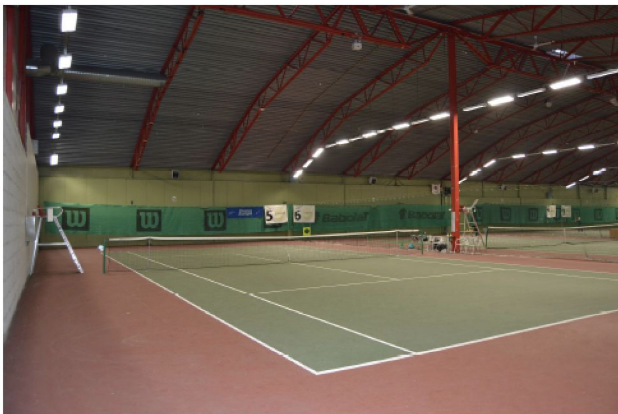
Ny LED belysning 8 baner Stavanger
